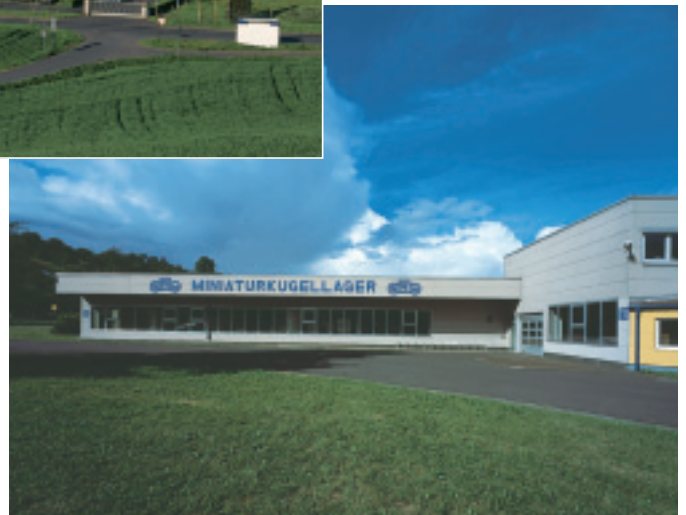
Rimpar production facilities
