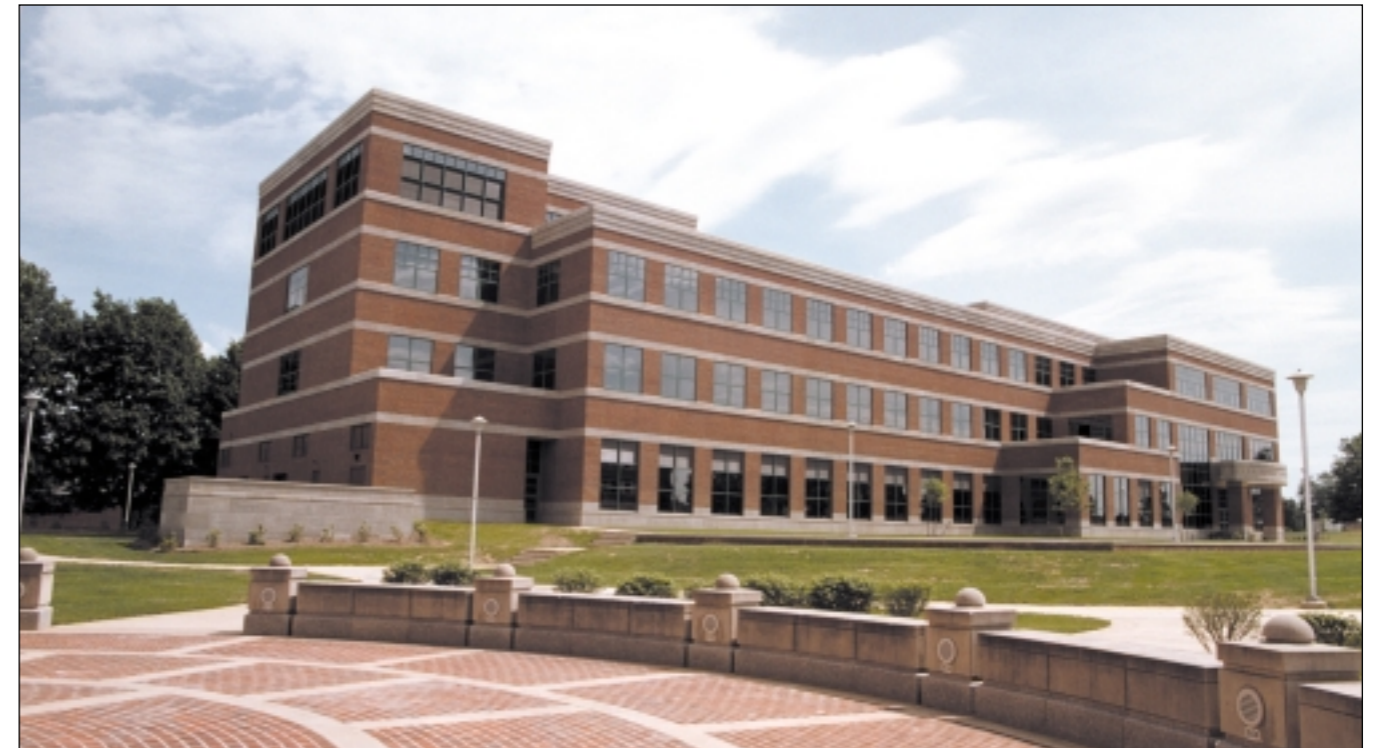
The recently completed Leonhard Building is home to Penn State’s Factory for Advanced Manufacturing Education (FAME), a state-of-the-art study facility that provides students with hands-on experience in a real-world manufacturing environment.
