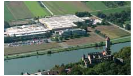
Werk Hassmersheim The FIBRO Hassmersheim plant Usine de Hassmersheim
