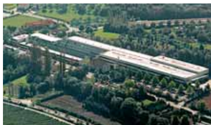
Werk Weinsberg FIBRO works at Weinsberg Usine de Weinsberg
