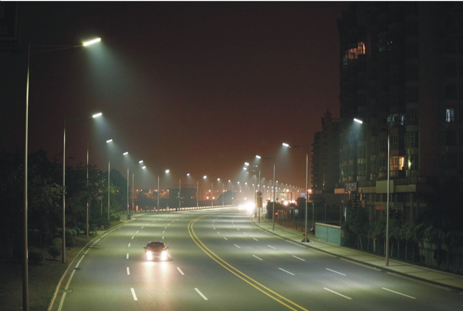
Street light project in Dongjiang road (6 lanes)
