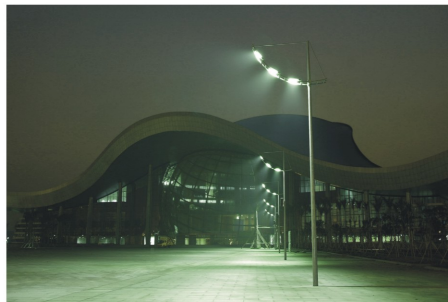
Street light project in Guangdong science centre
