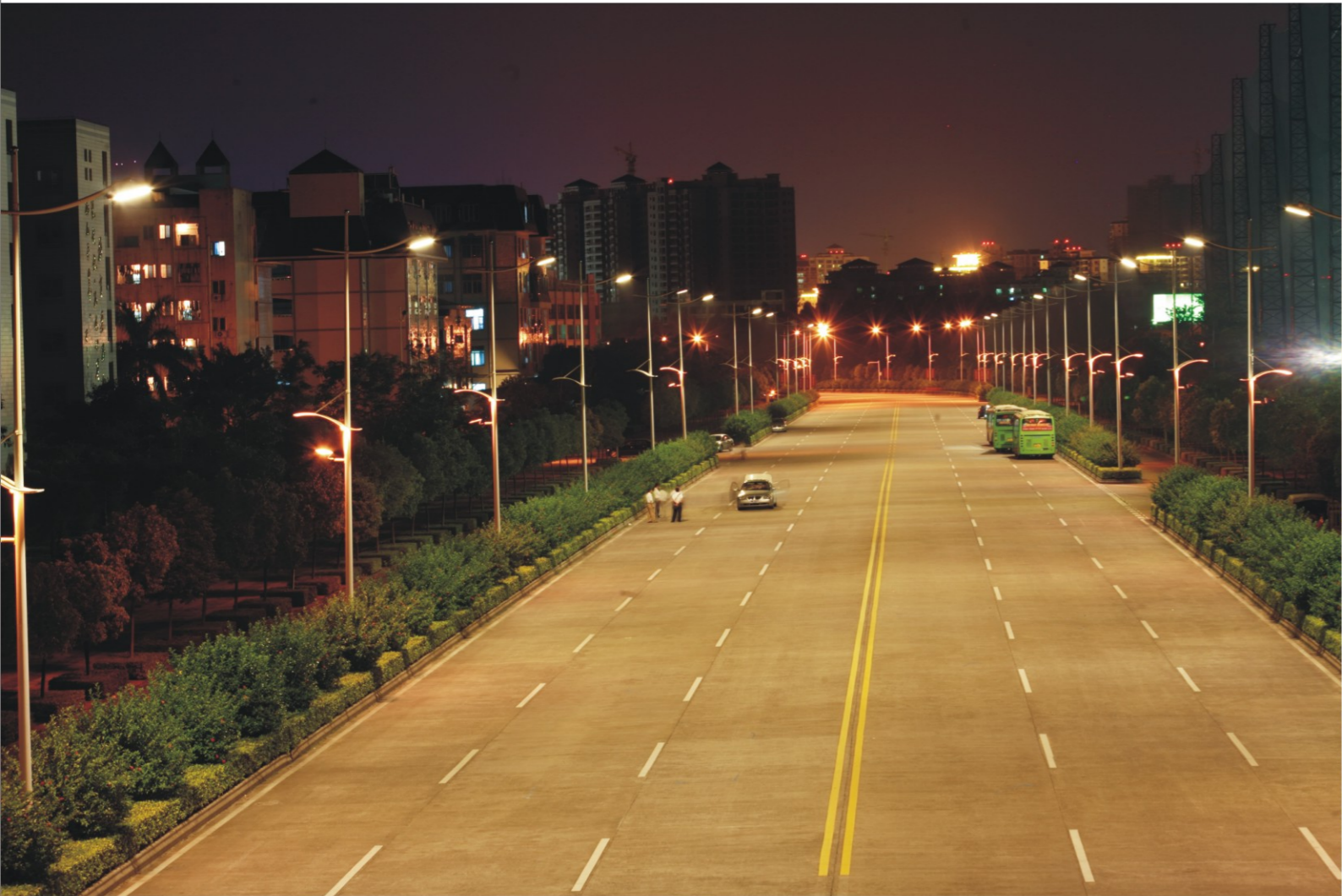
Street light project in Huizhou(6 lanes)
