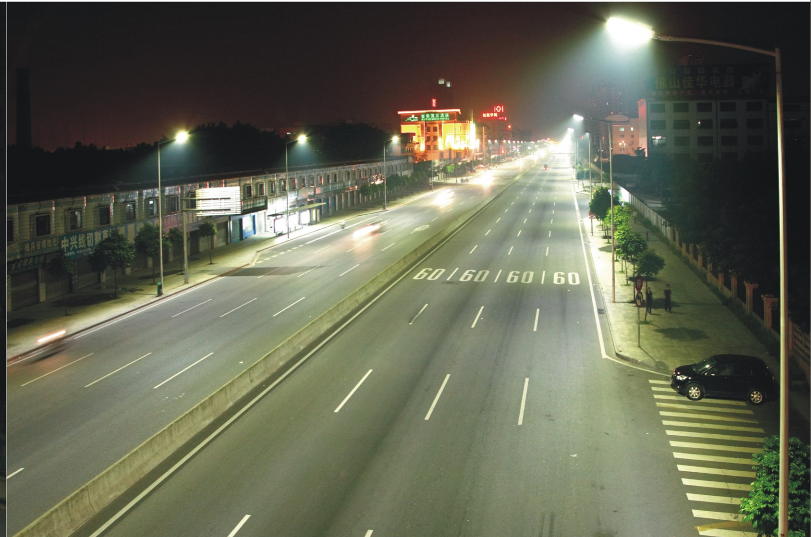
Street light project in Guanlong road (8 lanes)
