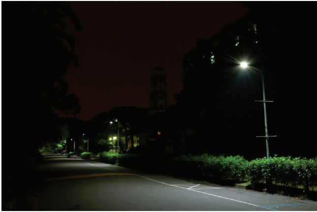
Figure 4. 200m roadway LED lighting field test in NTU.
