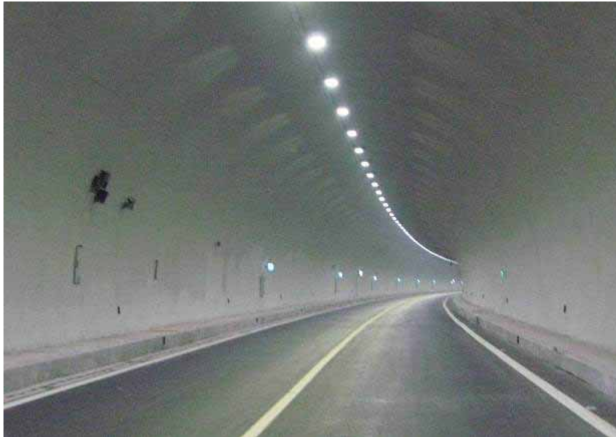
Zhangjiashan Tunnel on Chongqing Highway
