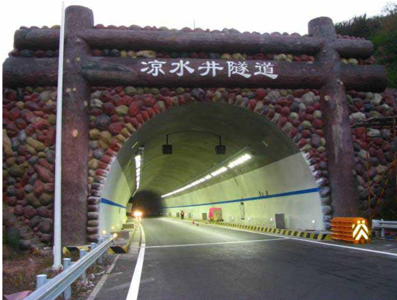
Hunan Province Chang Ji Highway Liangshuijing Tunnel
