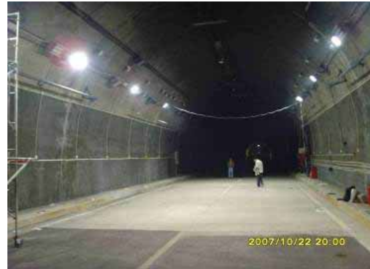
On Site Testing
