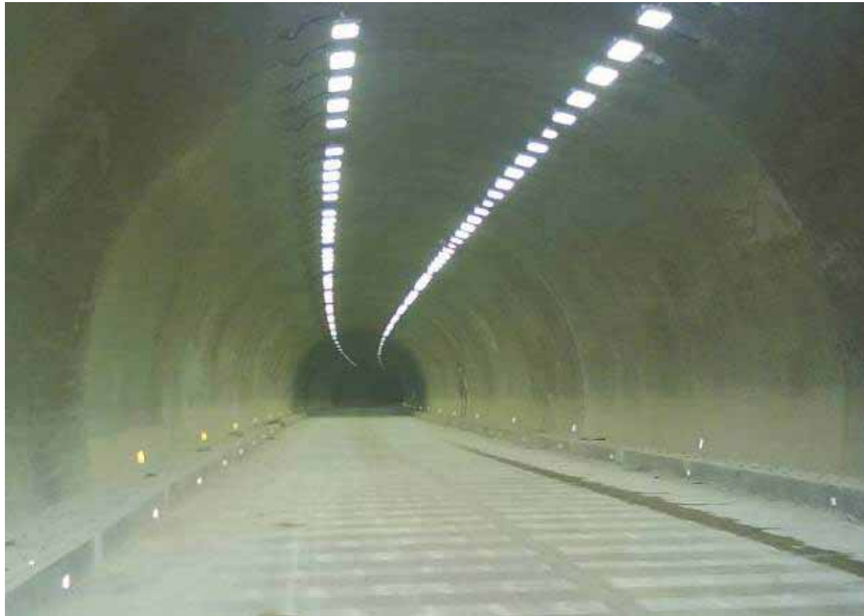
Fujian Quansan Highway Chaoyuan Tunnel, under construction
