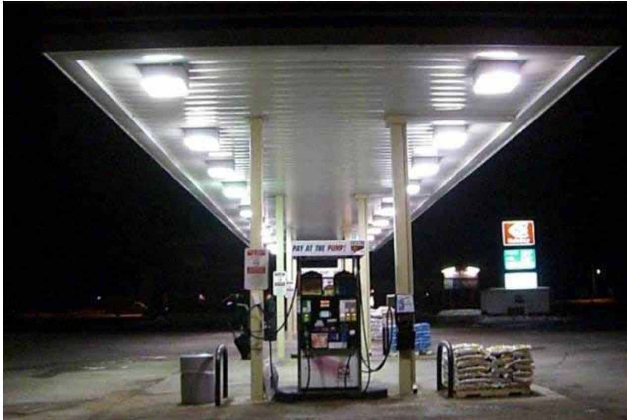
Gas Station Lighting, Minnesota, USA
