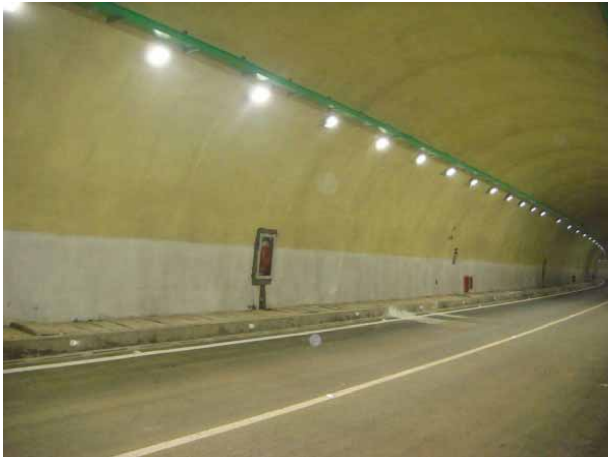
Jiangxi Jingde Town—Yingtang Highway Huangzhushan Tunnel
