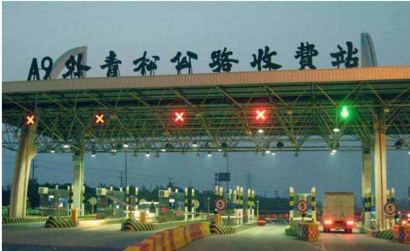
Shanghai Huqingping Highway Waiqingsong Toll Station
