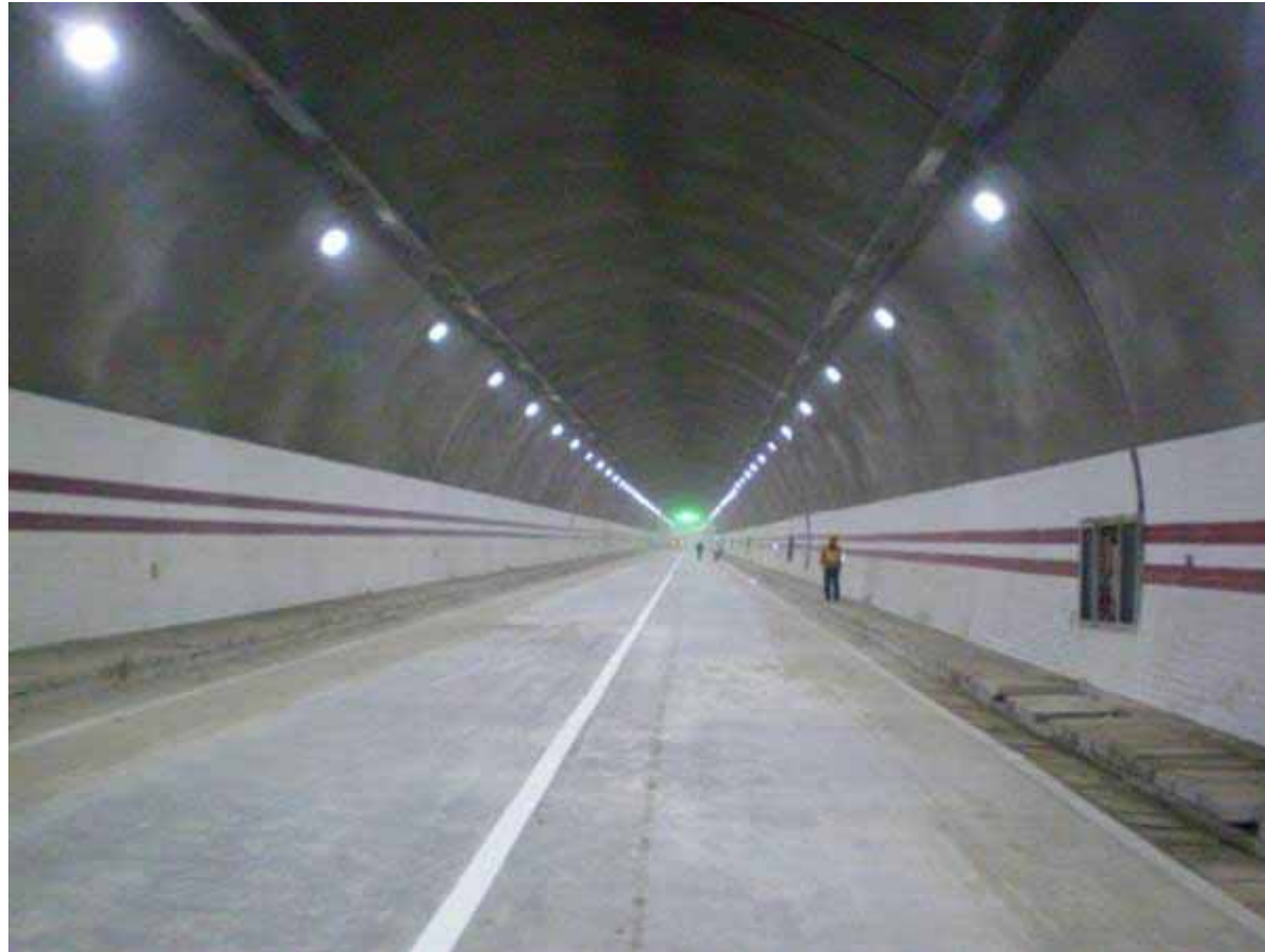
Yunnan Fuyan Highway Donglai Tunnel Left Bound Traffic
