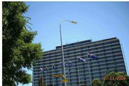
LED Street Light, LU6 in Australia
