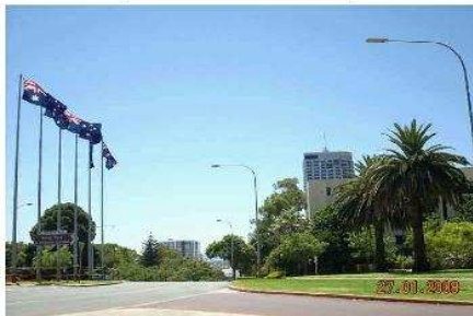
LED Street Light, LU6 in Australia
