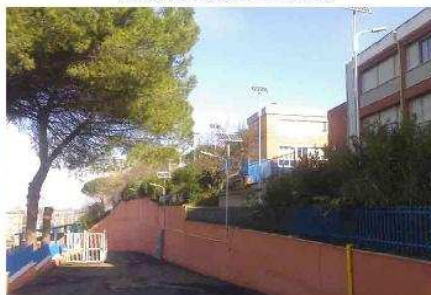
LED Street Light, LU2 in Italy
