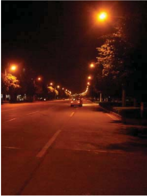
Before with HID luminaires
