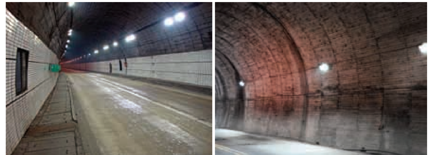
■ Tunnel detail, Taiwan
