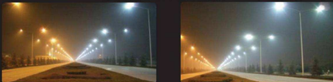
Left is 250w high pressure sodium lamp, Right is 60w LED lamp.Electricity saved more than 70%.
