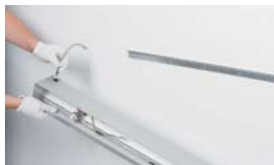
08 put wire through opening
