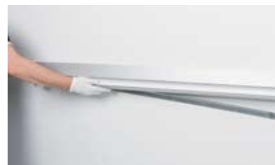
09 hang profile on the mounting rail
