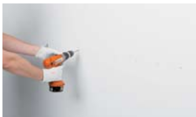
02 drill fixation holes on line
