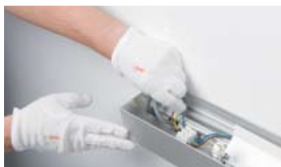
11 make electrical connection
