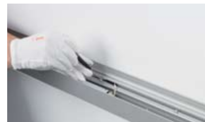
10 lock profile on rail by fixing the screws
