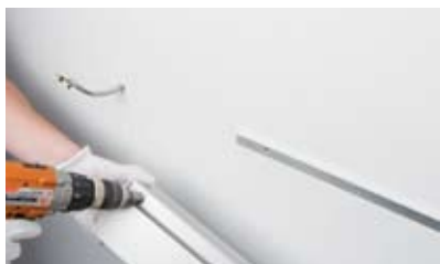
07 drill power feed hole in back of profile (min. 12mm)
