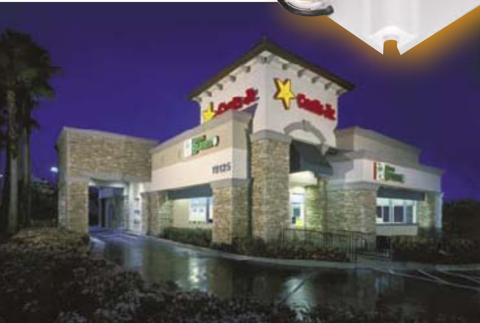
Figure 2. After an electrical fire destroyed the face of a Carl's Jr. fast-food franchise sign, the neon signage was replaced with new LED signage powered by Advance Transformer's signPRO LED drivers. Input watts dropped from 200W to 38W with the LED system, producing a payback of less than two years.
