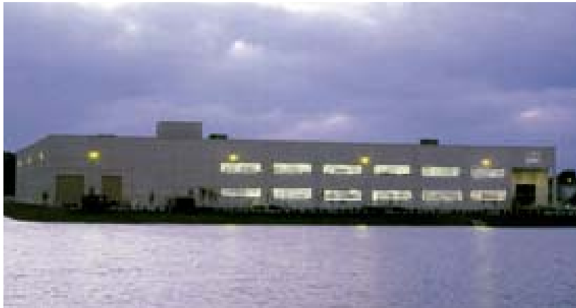
Super Vision's headquarters and 80,000 square-foot manufacturing facility in Orlando, Florida USA with 3,000 square-feet dedicated to an application showroom and classroom.
